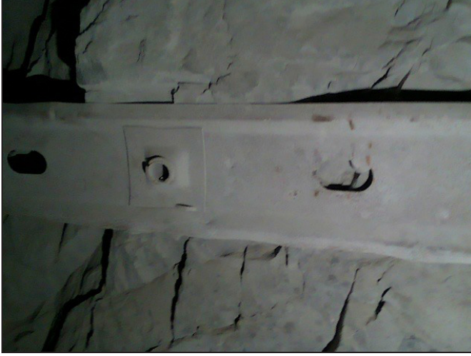
Figure 1. Shows a typical color image of the roof with a bolted strap, taken at the Edgar Mine in Idaho Springs, CO. It is imperative for any computer vision system to be able to differentiate between the strap and the underlying rock
