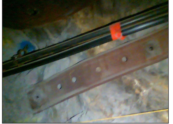
Figure 3. Shows an image of the roof from a typical point-of-view of a roof bolting drill. It is critical to be able to differentiate the strap from the rock
