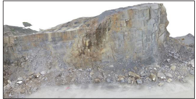
Figure 1. Highwall face looking at the east
