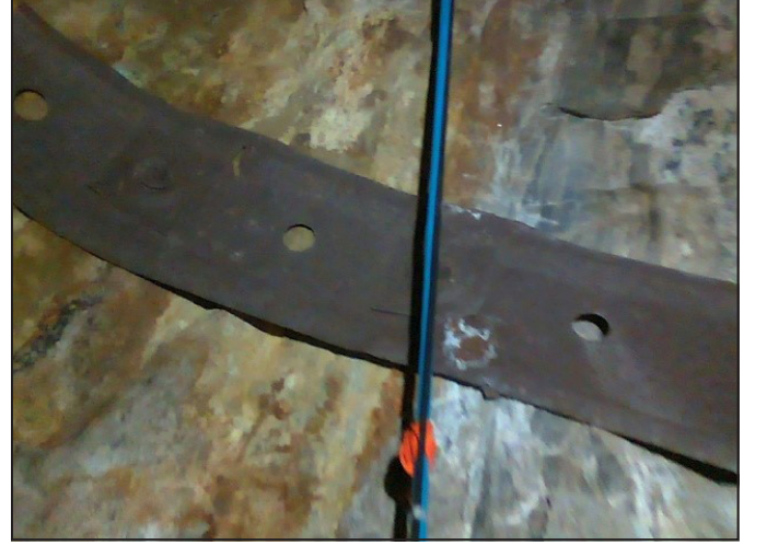
Figure 1. A scenario of rock, strap, and power cable area in the Edgar Mine in Idaho Springs, CO where it is required to identify the drillable regions from non-rock regions
