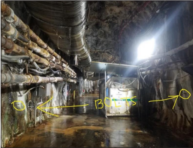
Figure 7. TPL2 or 68 level pump station area of bolt testing and overcoring in 2015
