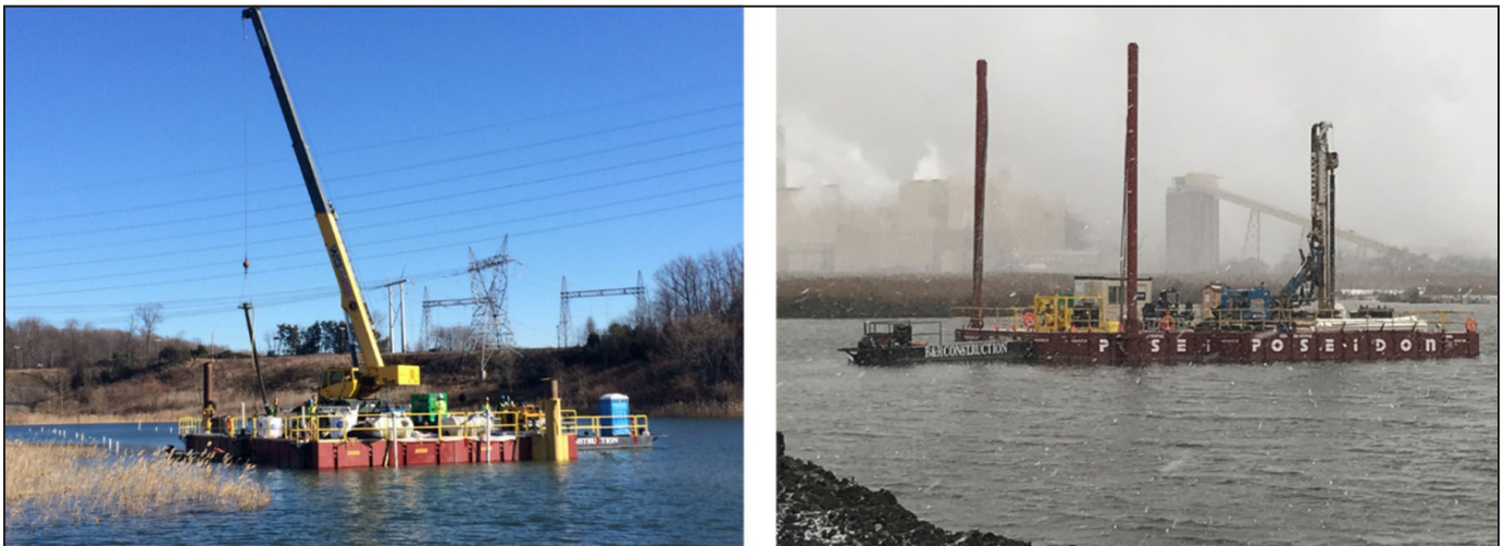
Figure 9. Floating equipment for well installation
