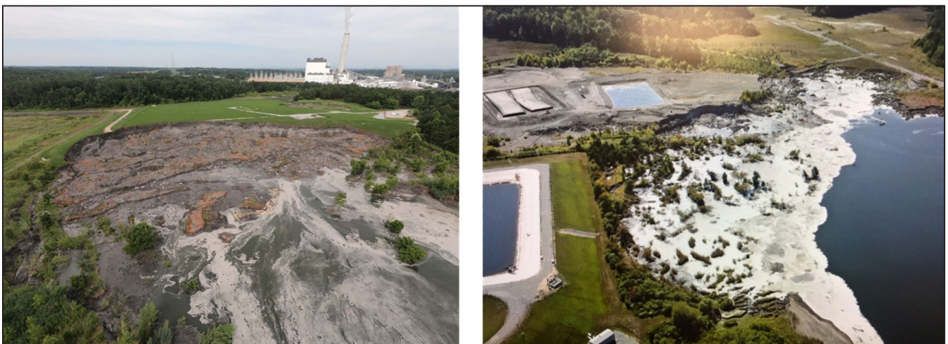
Figure 10. Examples of rapid drawdown failure
