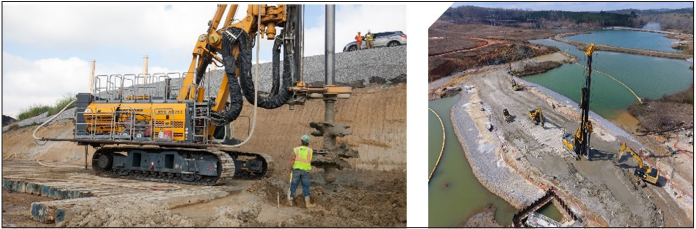
Figure 11. Soil mixing in ash
