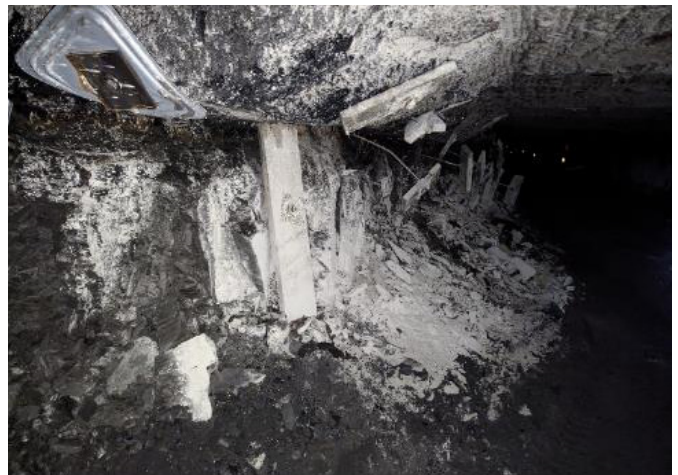
Figure 19. Example of rib sloughage, loose rib bolts, and the potential for brow formation of a coal rib
