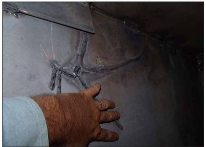
Figure 2. Fatigue crack repair
