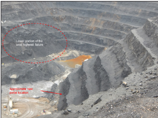
Figure 6. A view looking parallel to the highwall and catch benches above the proposed portal location
