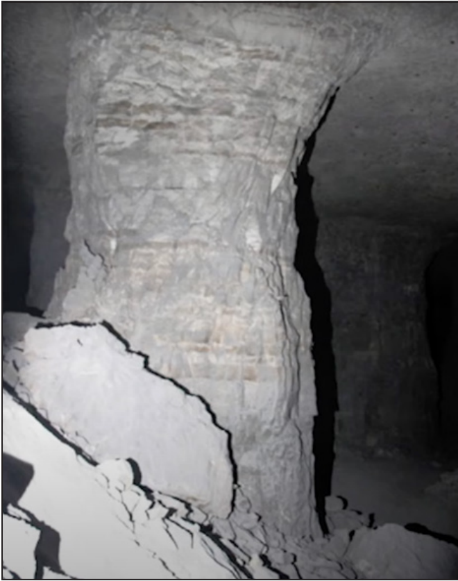
Figure 2. Hour-glass shape of pillars left after benching
