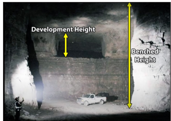
Figure 1. Typical large-opening stone mine with benching
