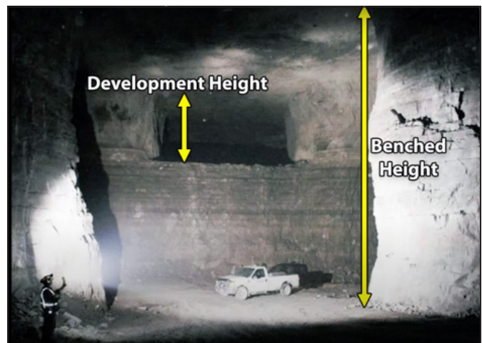
Figure 1. Typical large-opening stone mine with benching
