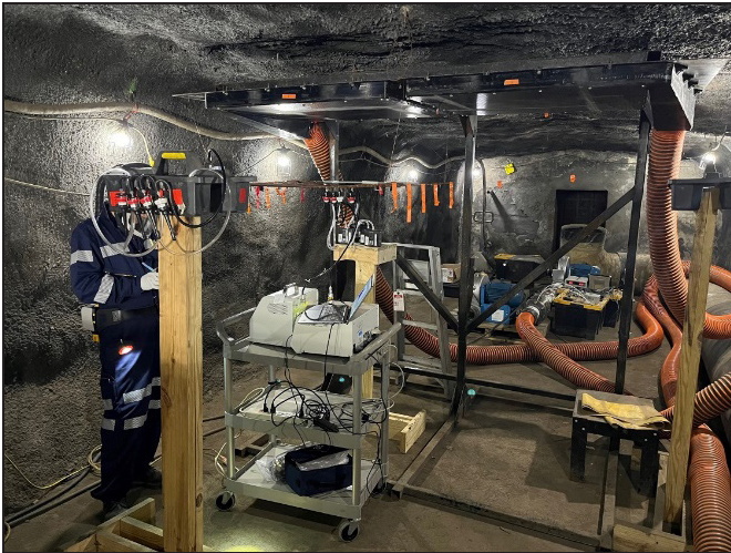
Figure 5. Photo of the DCAC inside the test entry showing the sampling baskets, real-time instruments and measurement grid
