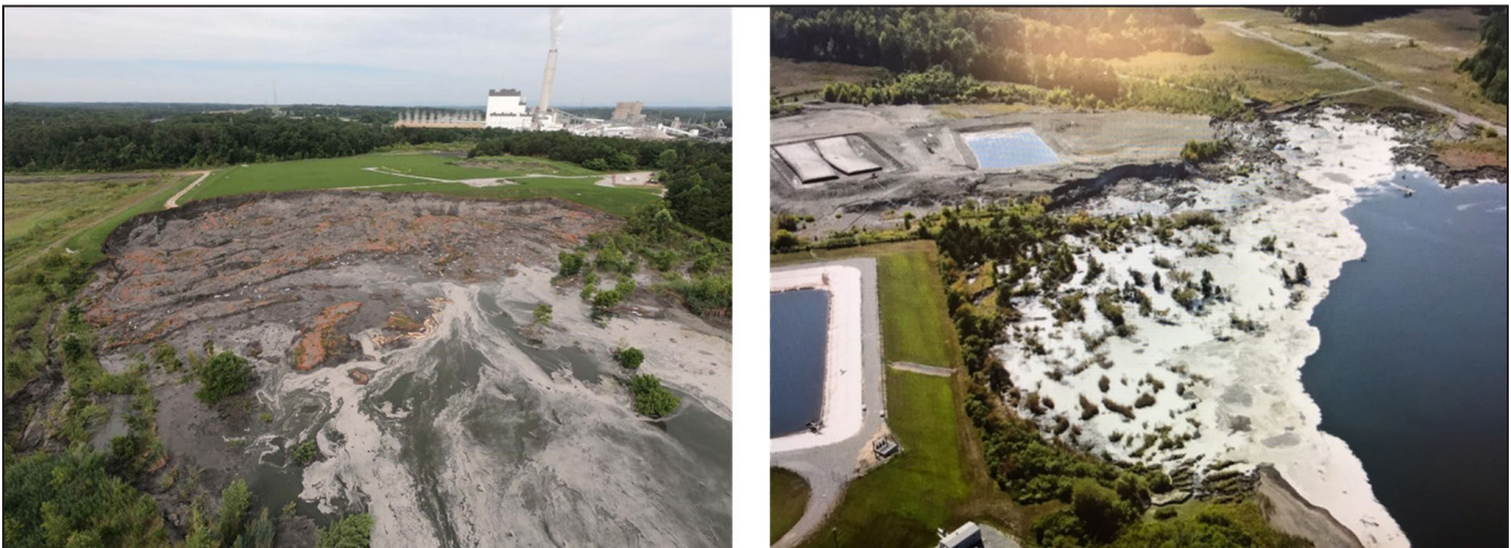
Figure 10. Examples of rapid drawdown failure
