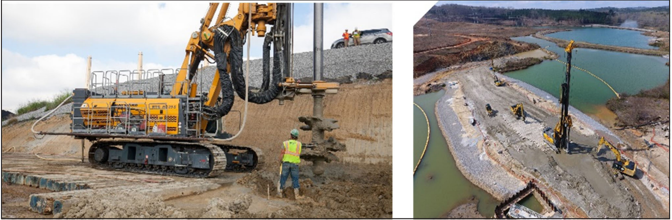
Figure 11. Soil mixing in ash
