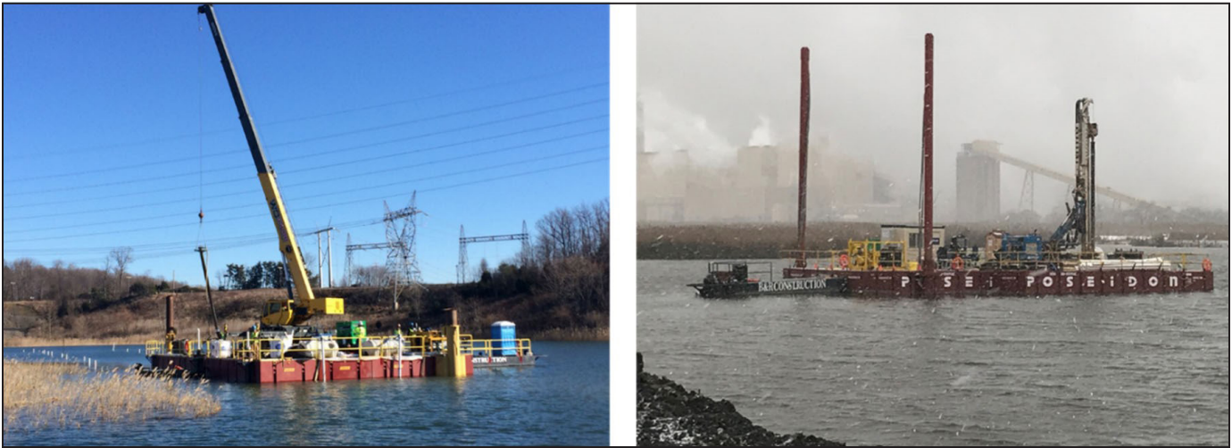
Figure 9. Floating equipment for well installation
