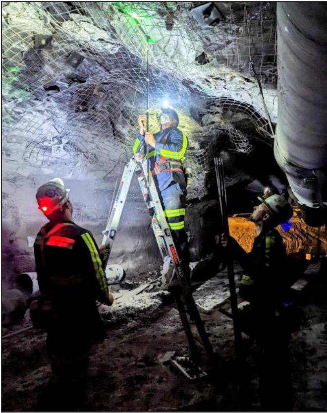
Figure 6. Photo depicting researchers safely using a ladder to install instrumentation
