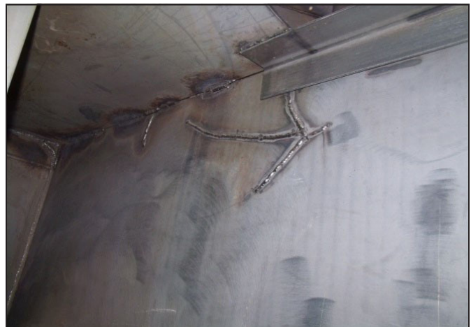
Figure 1. Typical fatigue cracking repair
