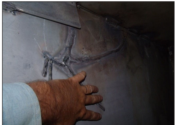
Figure 2. Fatigue crack repair
