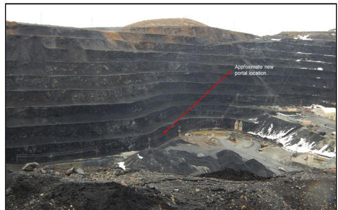
Figure 4. View of the highwall above the proposed portal location. The catch benches contain material along each bench toe; however, there are no signs of slope movement.
