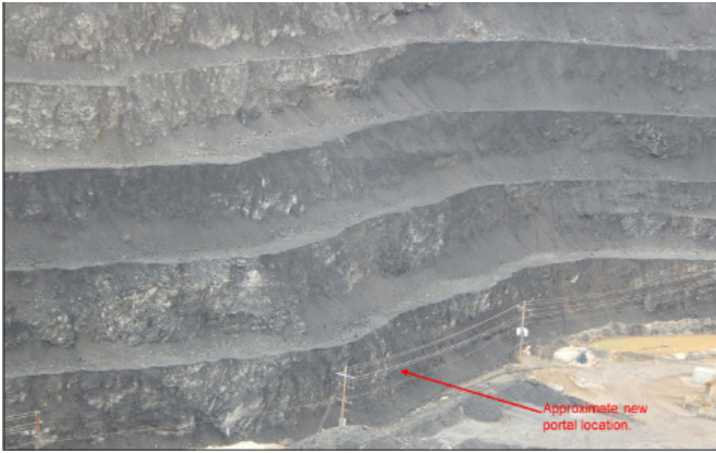
Figure 5. A closer view of the highwall above the proposed portal location
