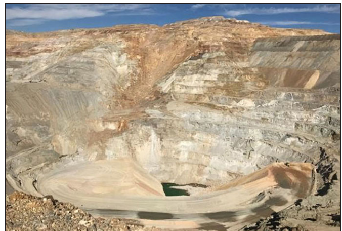
Figure 5. Photograph of the northern wall taken in 2020. Backfilling operations were started to buttress against further movement.
